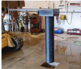
Place cylinder in hole.
