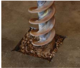
Auger hole for cylinder.
