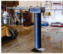
Place cylinder in hole.
