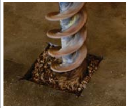
Simply saw through concrete. Auger hole for cylinder.
